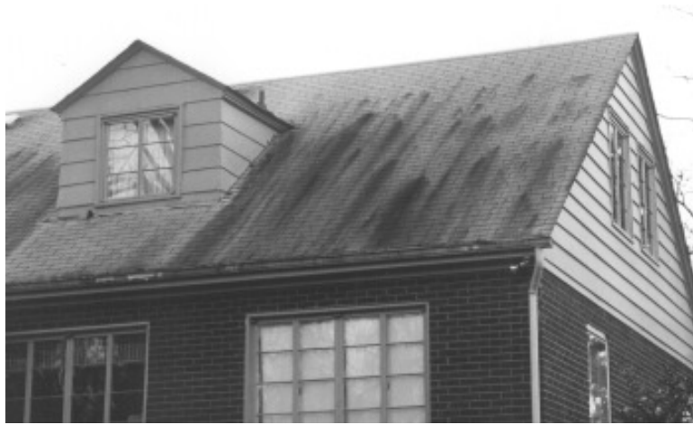
Figure 2. Mildew and algae on shingled roof.
